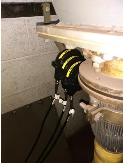
RFCTs fitted to cable earth strap
