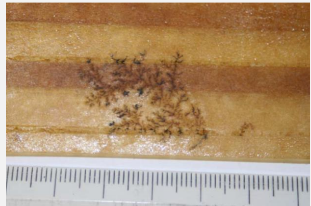
Paper Insulated Cable PD Damage
