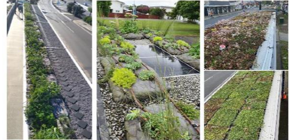
Figure 1: From left - Panmure Green Roof eco pillows; Diorella Drive roof with solar panels (Images courtesy of Auckland Transport); and Sempregreen Click'n go trays (Image courtesy of Greenroofs Ltd).
